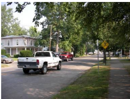
Crossing Sign Obscured and No Pavement Markings
