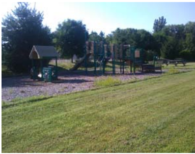
Replacing Mulch at the Playground at Karr Park
